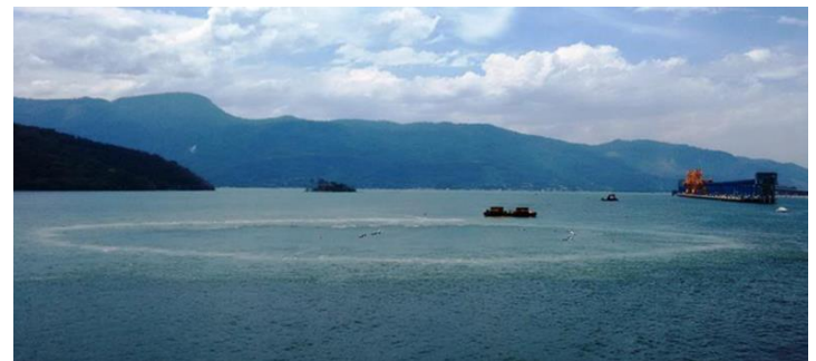
Fig. 10 Burble Curtain placed around of the blast area.
